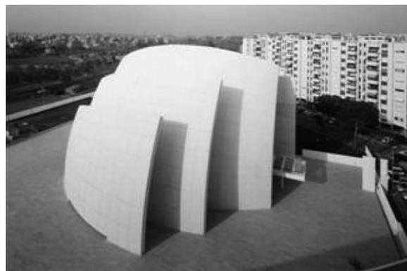
Fig. 13. The Dives in Misericordia Church, Rome, Italy. Outside surface of the church was coated by cement including  $\text{TiO}_2$  [145] (needs permission; directly cited).
