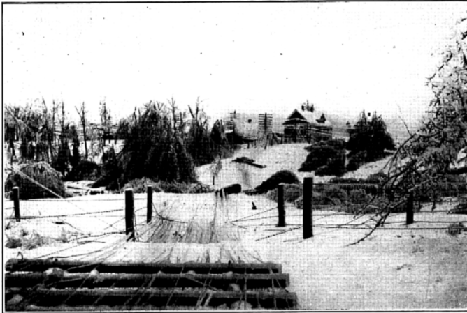
Fig. 3—Damage to Section of New York-Boston Main Line Near Worcester, Mass. Storm of November 28, 1921
